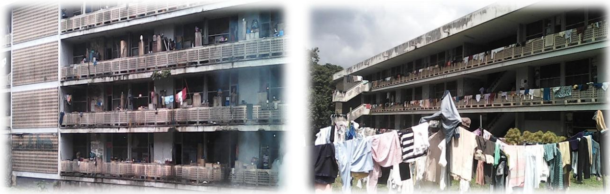
Figure 2a; 2b: Discoloration in Building
