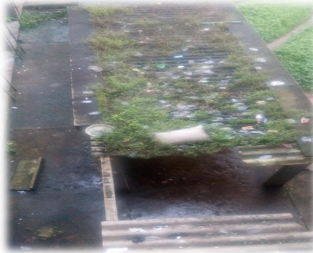
Figure 4: Crack in Roof
