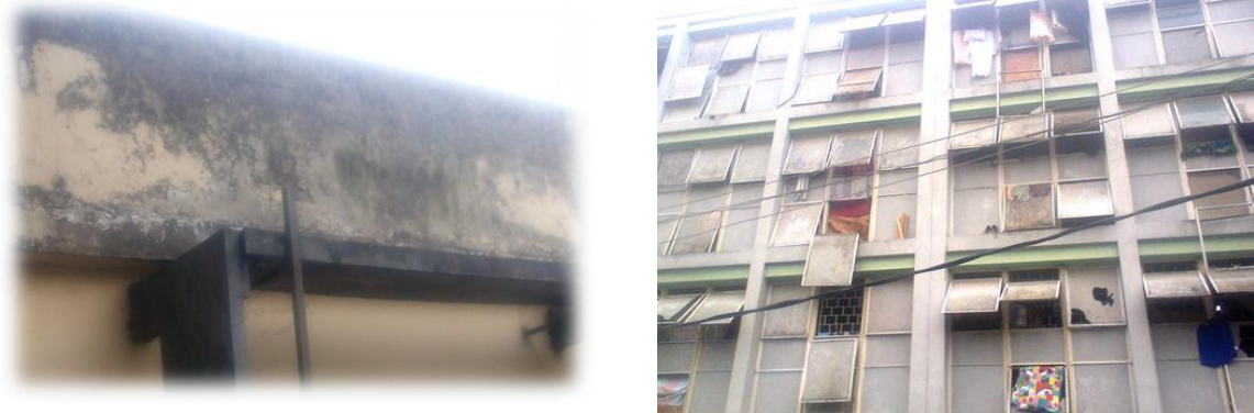
Figure 1a: Peeling and Cracking in Paint and Glass
