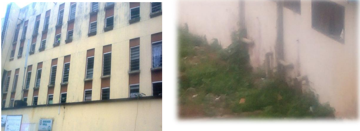
Figure 1b: Penetrating Damp on the Wall
